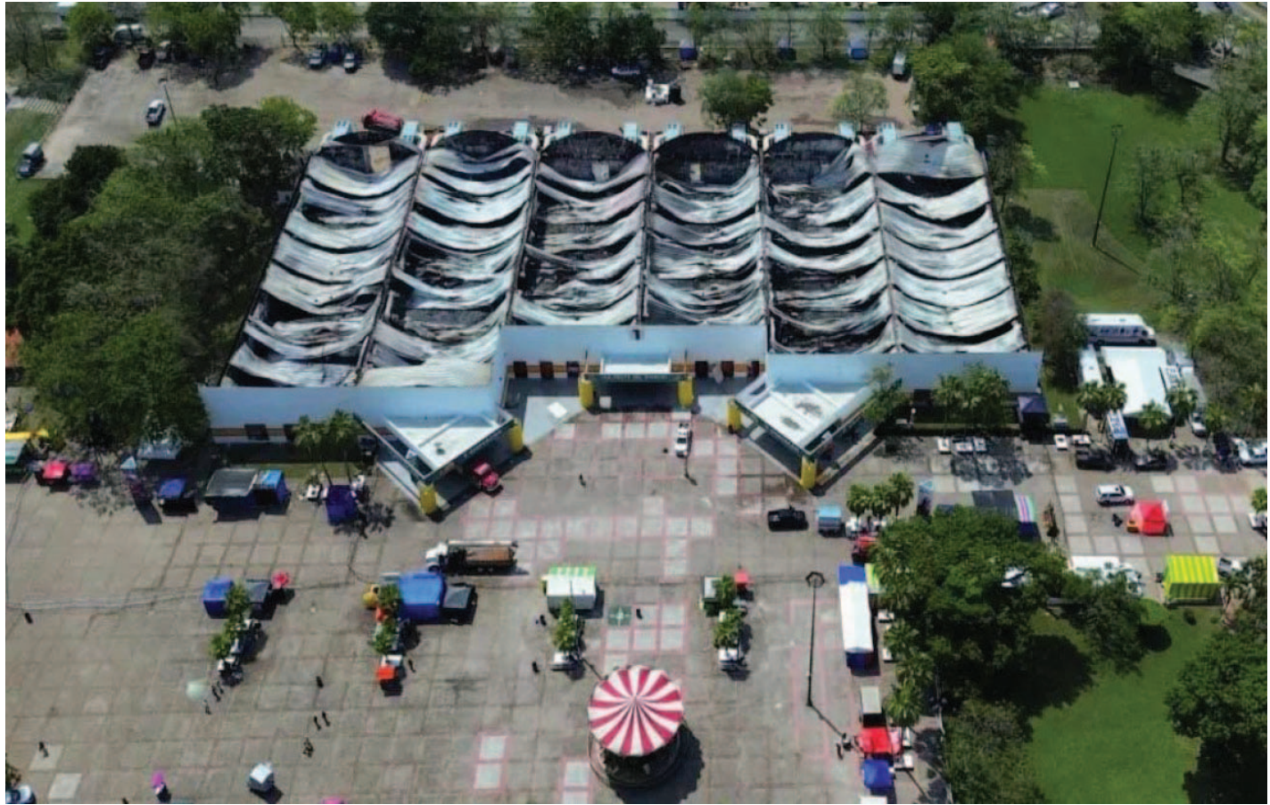
Reuters A drone view shows the aftermath of a deadly fire at a fairground in Mexico's south-eastern city of Villahermosa, Tabasco state. Photo: 7 May 2026 Reuters
