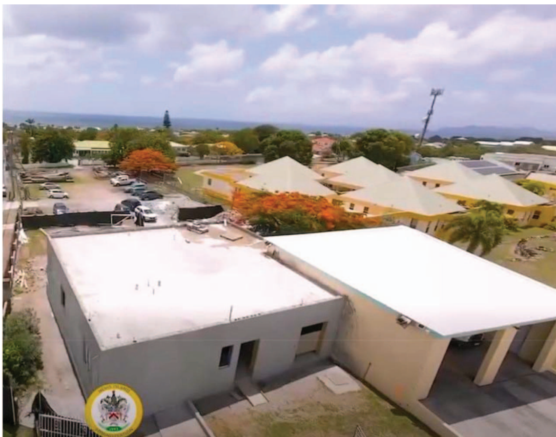
Nevis Island Administration constructing Nevis' first-ever Dialysis Unit at the Alexandra Hospital
