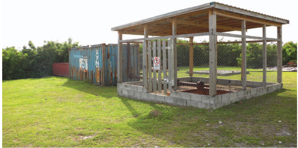
Nevis Geothermal Project well at Hamilton
