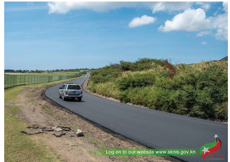
A section of the newly paved road
