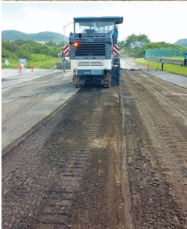
Nevis Public Works Department personnel and equipment deployed to assist on the St. Peters Road Rehabilitation Project in St. Kitts
