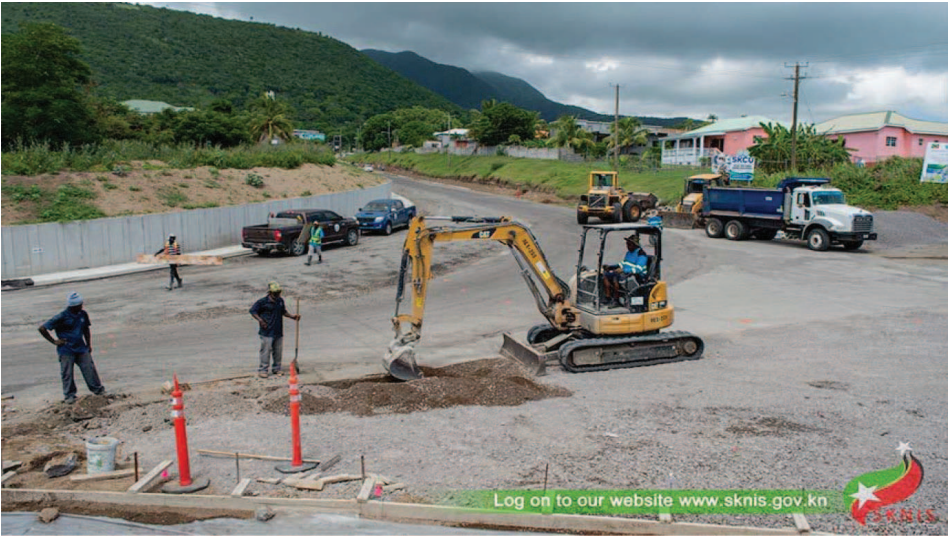
The new St Peters Roundabout under construction
