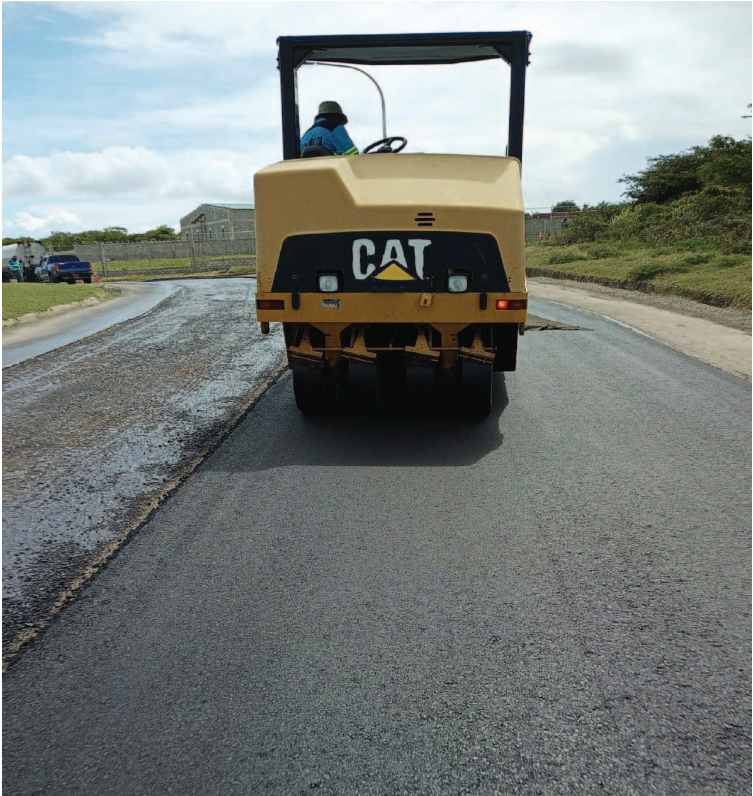
Nevis Public Works Department personnel and equipment deployed to assist on the St. Peters Road Rehabilitation Project in St. Kitts
