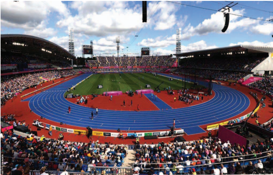
General view of the Alexander Stadium in Birmingham during the 2022 Commonwealth Games
