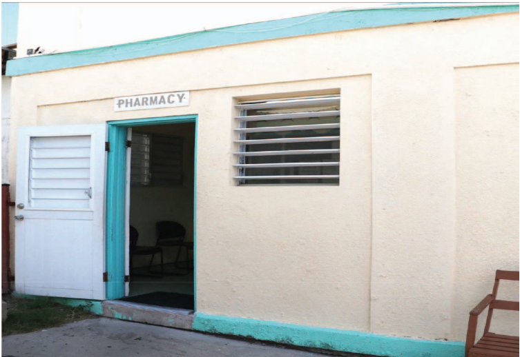
Pharmacy facility at the Alexandra Hospital, Nevis
