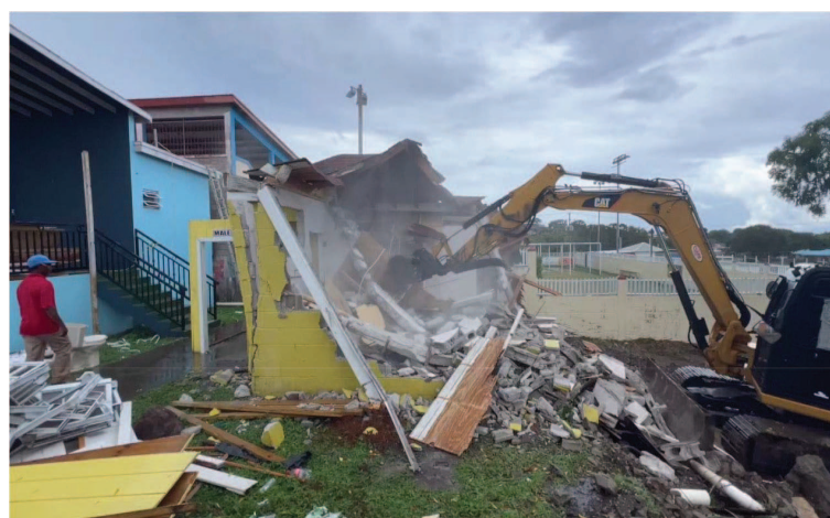
Nevis Cultural Village undergoing renovation and upgrade
