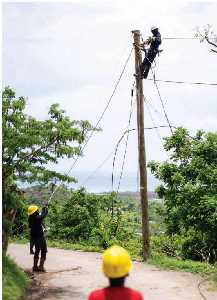
NEVLEC lineworkers among crews working to help restore electricity on the storm ravaged island of Carriacou
