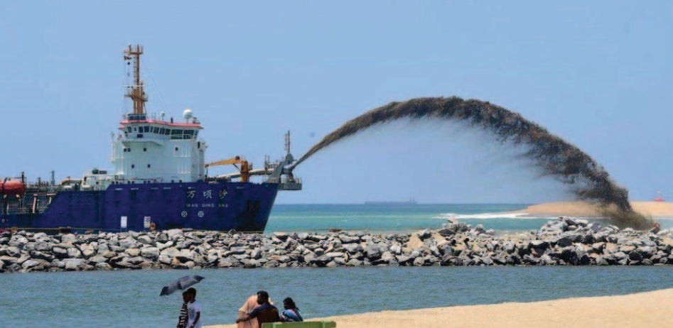
A dredger pumps sand to reclaim land just outside the port of Colombo in Sri Lanka in 2017 IMAGE SOURCE,AFP VIA GETTY IMAGES A dredger pumps sand to reclaim land in Sri Lanka
