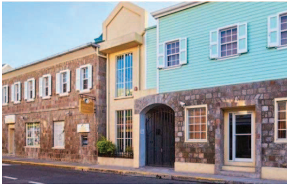
Headquarters of the Bank of Nevis Limited, Charlestown, Nevis
