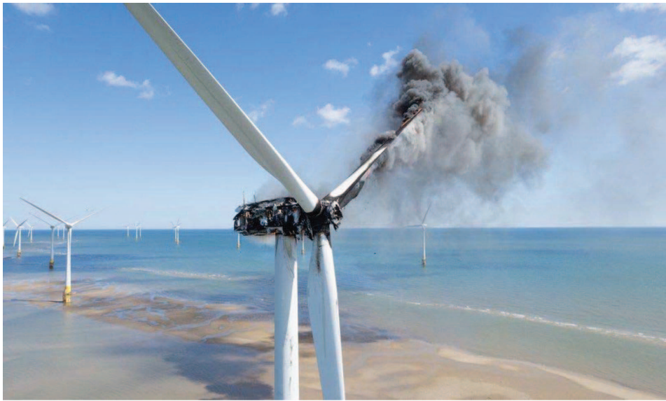
Smoke billowing from a wind turbine off the coast of Great Yarmouth IMAGE SOURCE,OLIV3R DRONE PHOTOGRAPHY The turbine is part of the Scroby Sands offshore wind farm
