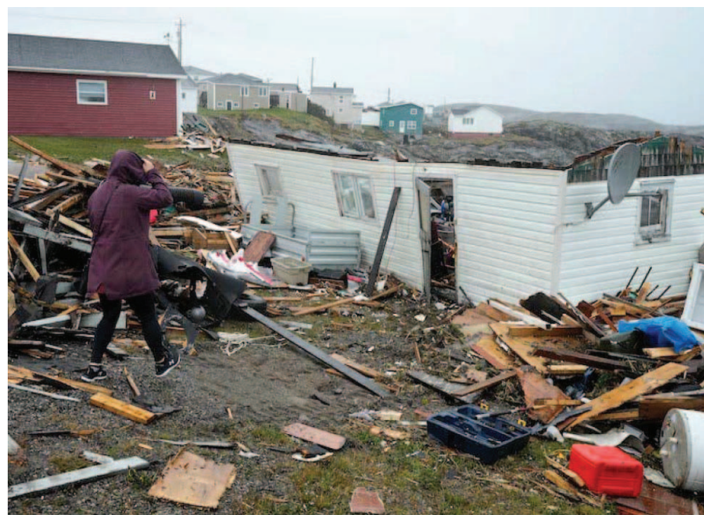
A resident approaching the destroyed remains of a home in Port aux Basques, NL. Photo credit: Frank Gunn (The Canadian Press).
