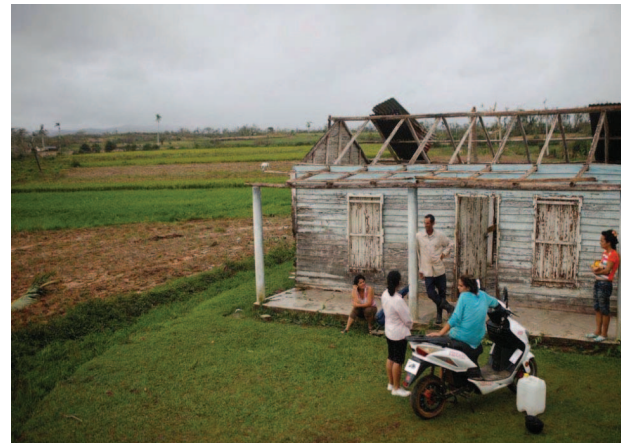
A family gathering in front of their destroyed home in the aftermath of Hurricane Ian in El Cafetal, Cuba, 27 September 2022. Photo credit: Alexandre Meneghini (Reuters).
