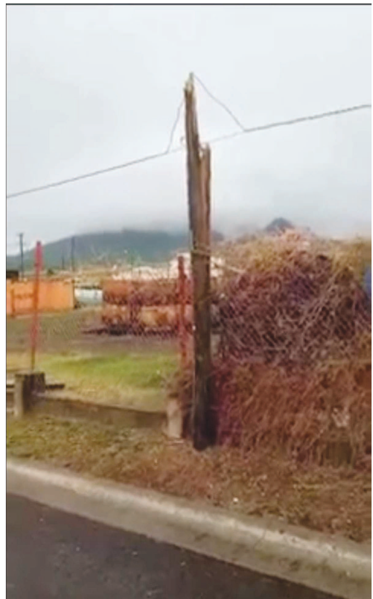
Photo: A video screenshot of the damage electrical pole damaged after being struck by lightning in the Lime Kiln community on Wednesday 30th June 2021
