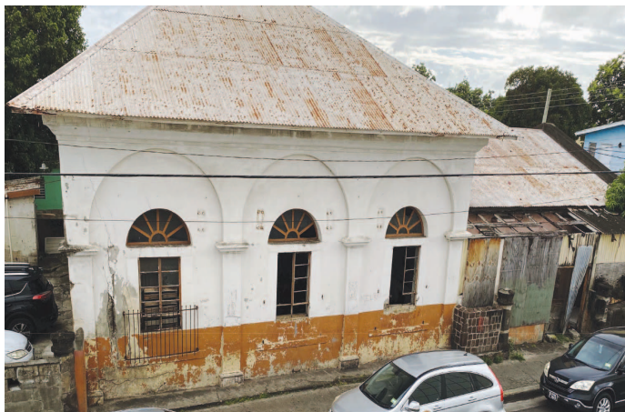
Old Ice Plant Building
